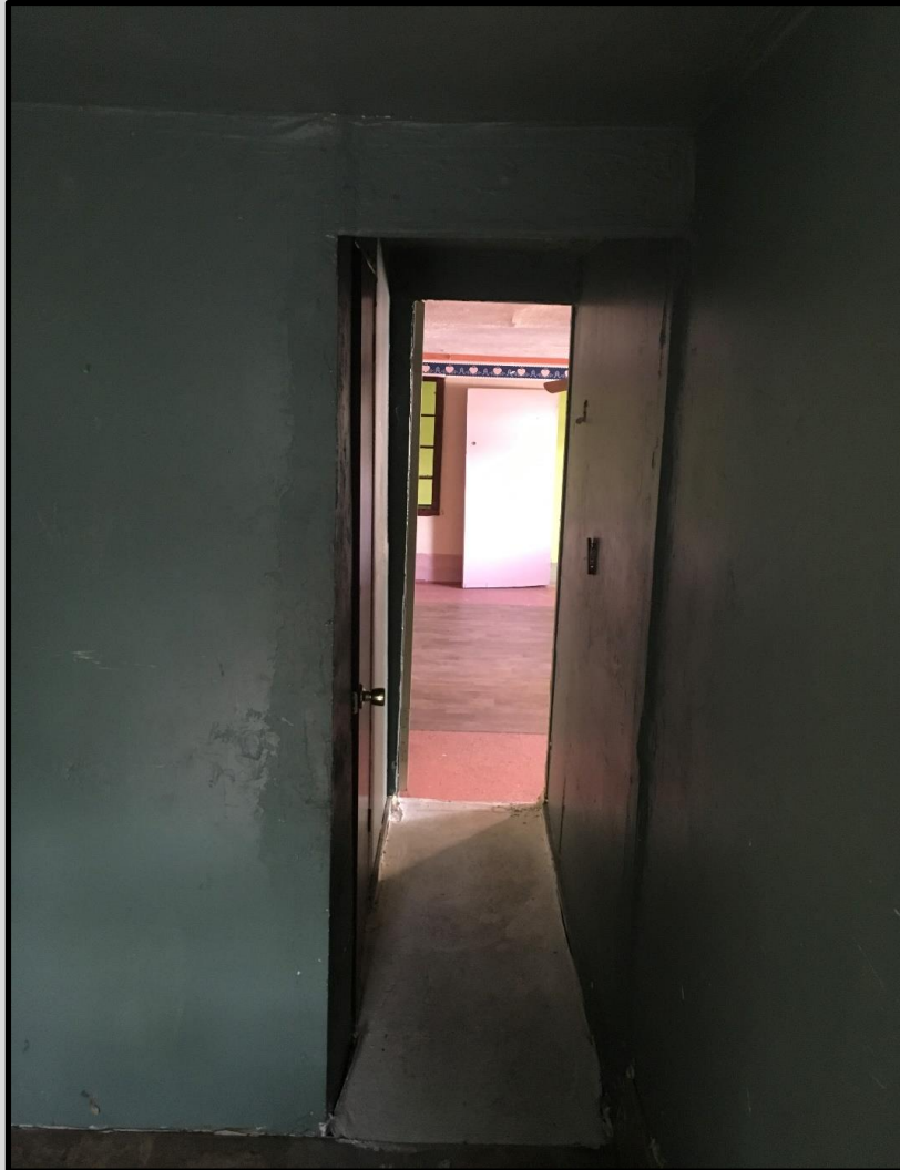
June 29, 2018 Inspection Pictures 2020 Dixie Avenue Case #17-00911
