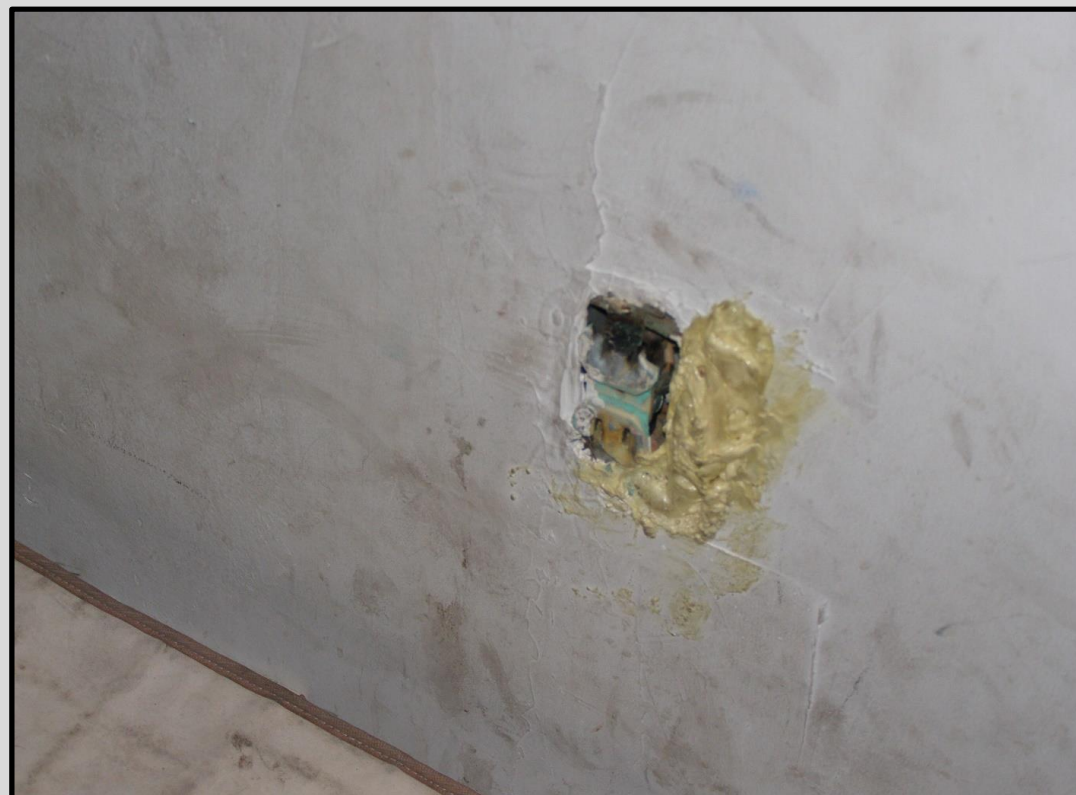
Electrical/fire hazard
